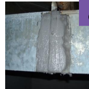
Seal ducts, blow insulation
