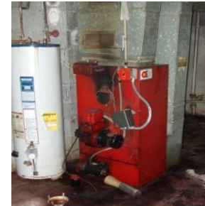
Broken hot water heater and furnace
