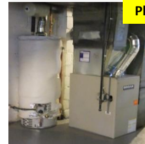
Install furnace and hot water heater
