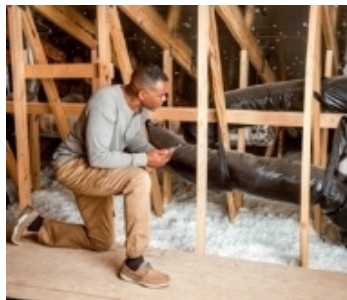
Attic & Wall Insulation
